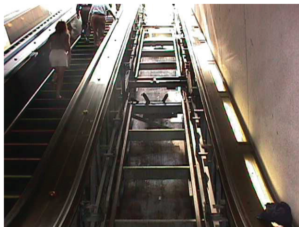
An escalator under modernization
