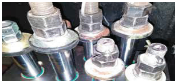
Figure 7: (top to bottom) A fixed dynamic load adjusting system (hydraulic), pictures of Henning Rope Harmonizer systems installed and an installation in the U.S.
